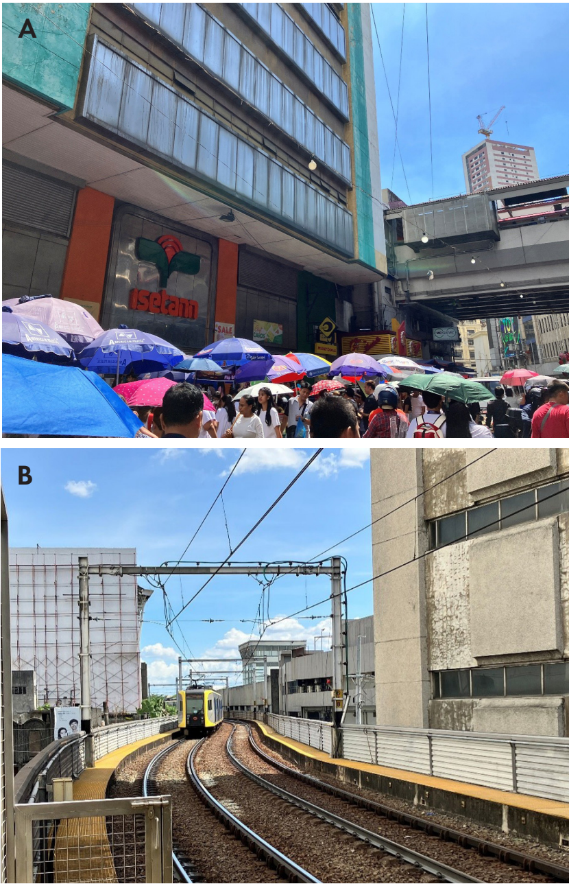
FIGURE 1. A, the Isetann Department Store, rebuilt to give way for the LRT-1. The LRT-1 Carriedo station is situated to the right of the image. B, the LRT-1 tracks looking south from Carriedo station. Note the narrow clearance between the buildings and the viaduct. Images taken by the author on May 2, 2025.
